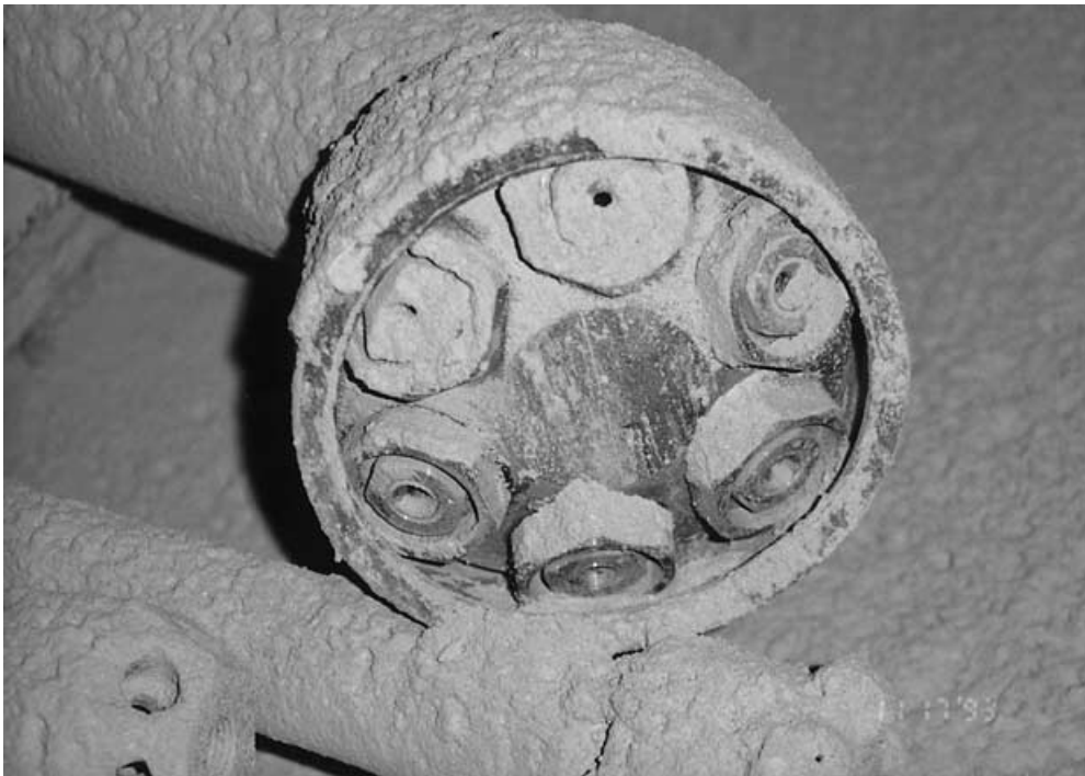
Figure 12.9 Close-up view of spray nozzles on end of water injection cooling lance.
